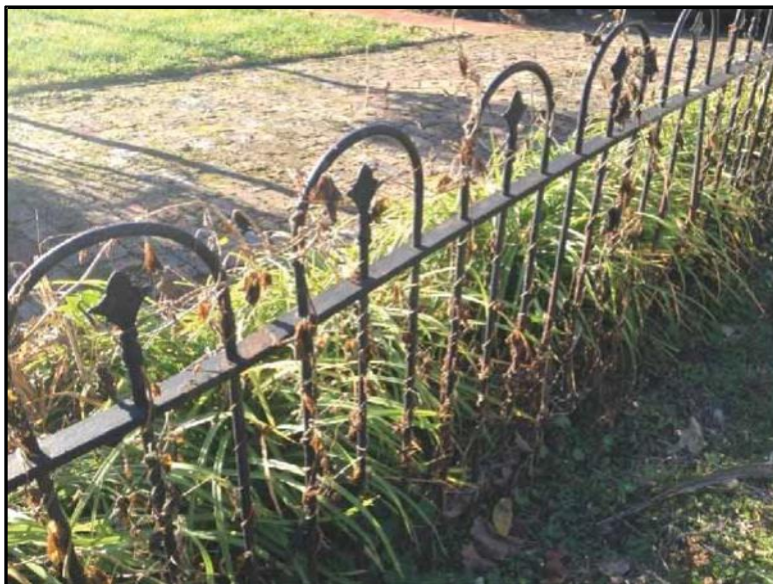
This decorative cast-iron fence will need a new protective coat of black paint to prevent further deterioration.
